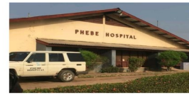
Supporting Phebe Hospital Isolation Units in Gbarnga, Liberia
